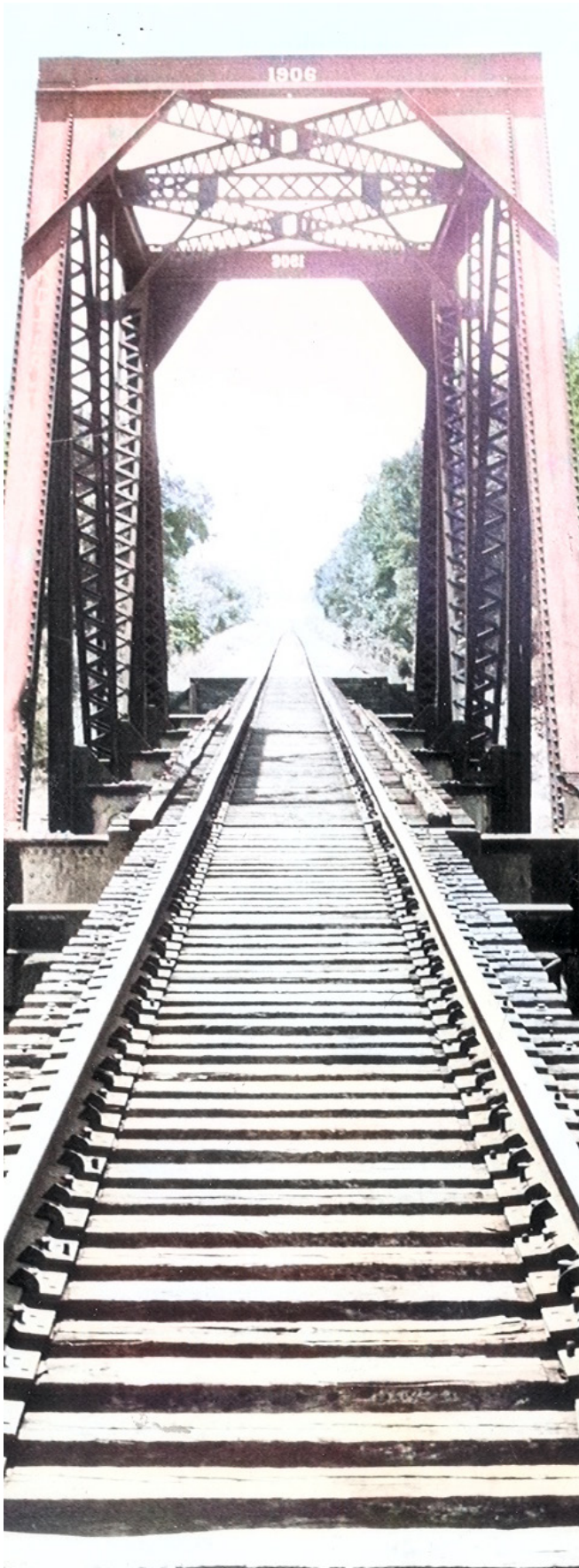
View of the old 1906 railroad bridge. Originally built in 1885, the bridge was renovated in 1906. In 2021, Union Pacific replaced the wooden trestle bridge with a concrete bridge, but retained the 1906 iron truss.
