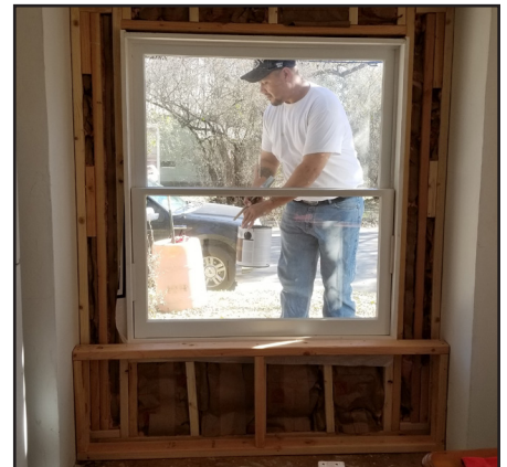
The 1900 Gaulden-Baskin House was awarded a $14,268 grant to replace six deteriorated aluminum windows with new wood ones.
