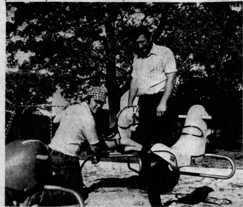
ALL WORK AND NO PLAY? — Park board member Joe Baker is helped by Phil Sutton in installing a piece of playground equip-
