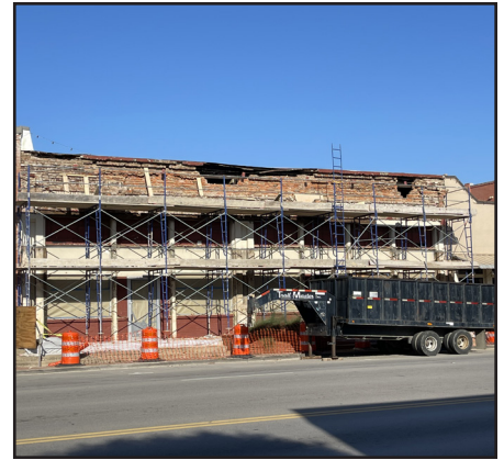
The 1890 Dennis Mahoney Building was awarded a $25,000 grant to restore its historic storefront.
